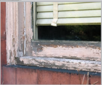
Old windows that have significant decay may be the perfect candidates for a Full Frame Replacement System, shown here.
