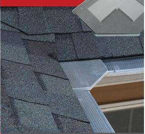
High volumes of water can overwhelm gutters in certain spots such as inside roof valleys. An inside roof valley is the point where two rooflines meet forming a 90° angle. This creates an inside corner with more water flow than any other area of the home and this increased volume always overshoots the gutter.
